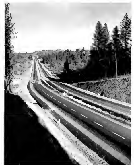
US 40 expressway through Sierra Nevada foothills east of Auburn
